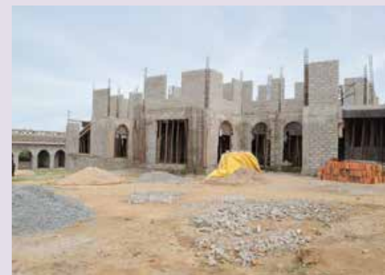
Construction progress of Rakai High Court and Chief Magistrates’ Court.
